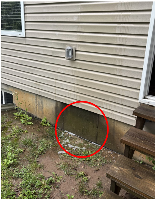
Water pooling next to foundation.
