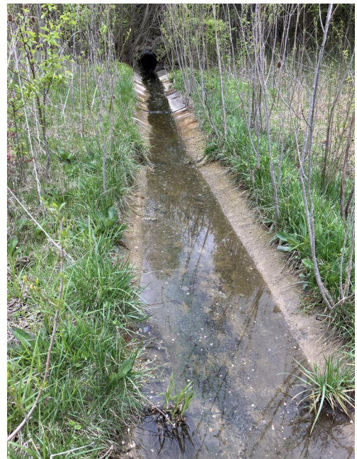
Private drainage easement, concrete lined.
