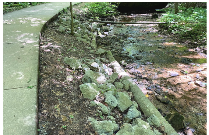
Toe Wood streambank stabilization.
