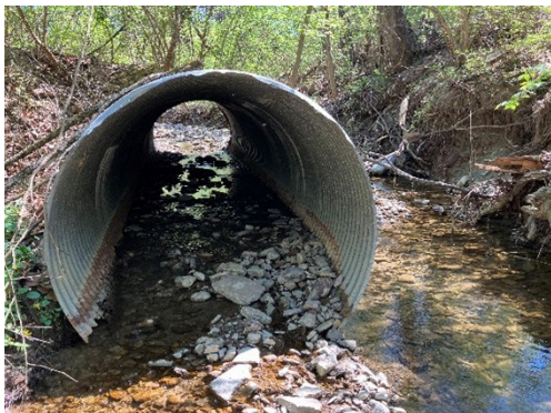
Stream eroded around culvert.
