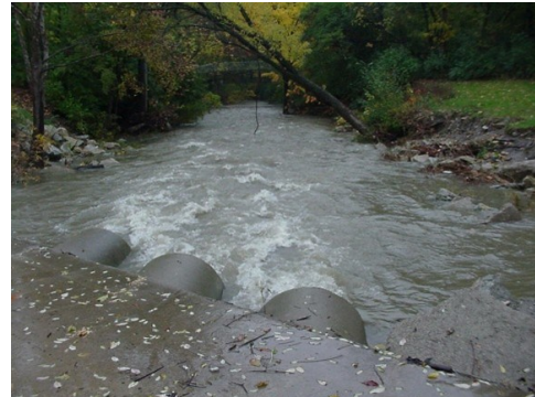
Shallow crossing on a stream reaching high velocity.
